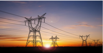
Electric T&D Infrastructure
